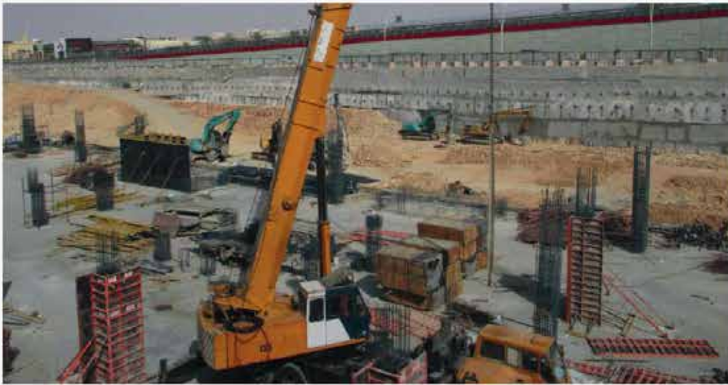
Suleiman Habib project site-King Abdullah Road
